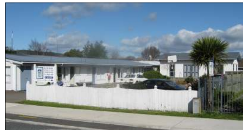
Picture of flats from outside
